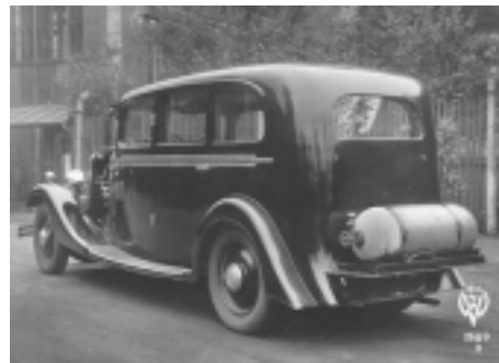
Czech passenger car Wikov running on compressed town gas – around 1936
