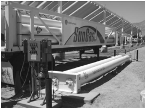
**Figure 3. SunLine's FIBA tube trailer and ASME tanks for CH<sub>2</sub> storage**
